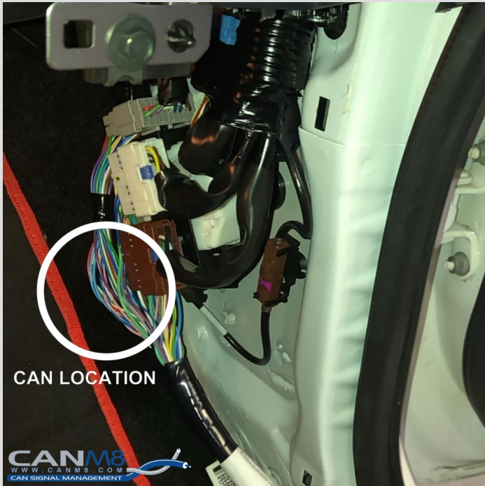
CAN wiring in the right side kick panel harness
