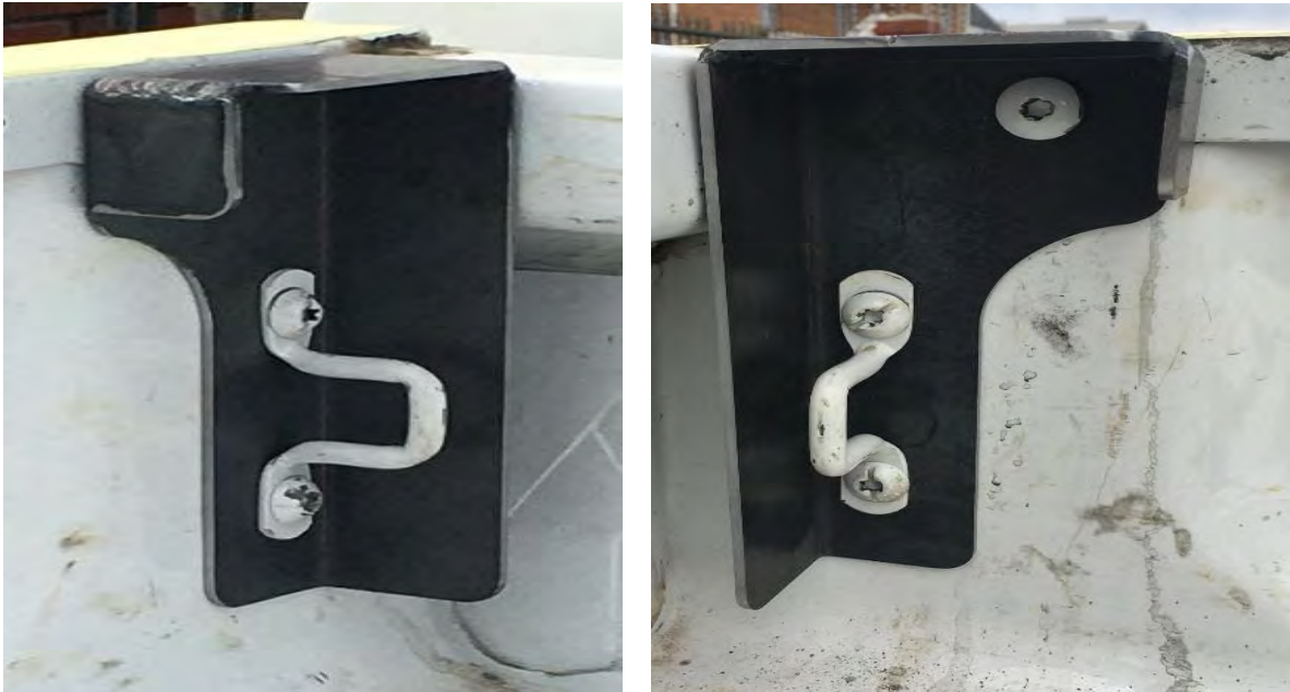
Figure 12: Front Bracket installed
